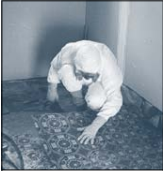
Lift and Peel up Flooring
