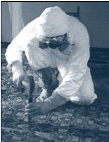
Cutting the Floor
