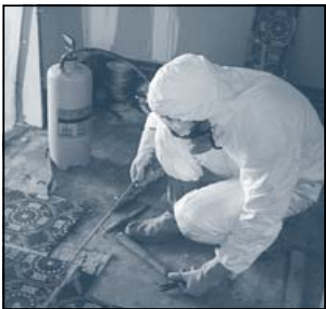
Wet the Floor Before, During and After Removal.
