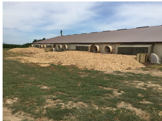
Figure 2.7 A flat open bed biofilter.
