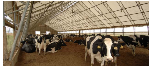
Figure 2.3 A hybrid-ventilation dairy barn.
