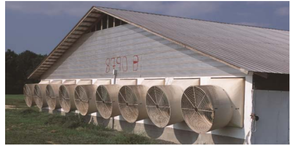
Figure 2.1 A mechanically-ventilated production house with ventilation fans.
