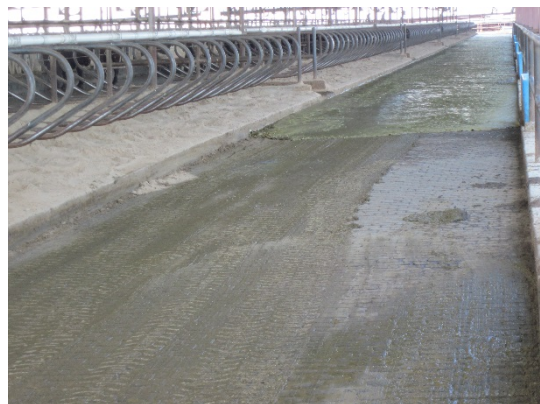
Figure 3.3 Flushing to remove manure.
