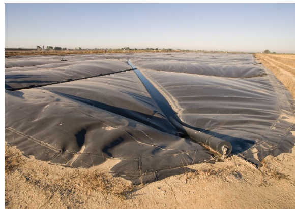
Figure 3.7 Covered lagoon anaerobic digestion in California.
